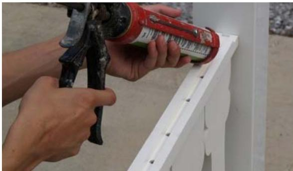
To install the top railing for a section, apply a bead of adhesive down in the groove on the top of the baluster assembly. Set the top rail in place making note that there are no big gaps or unevenness. Follow the same cleanup guidelines as provided for the bottom rail
