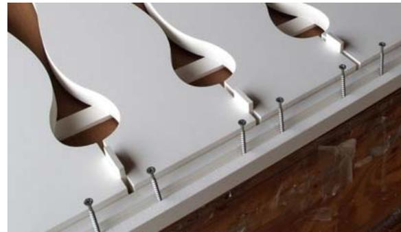
Drill holes larger than the body of the screws you will use to attach the Cap Rail to the Balusters. The screw threads should fit into the hole easily but not be too loose.
