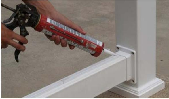
From experience, it is best to assemble the baluster sub assembly and the railing by installing the bottom rail first. Place shims every 24 inches under the installed bottom rail to prevent any sagging while assembling the baluster assembly and top railing. Apply a 3/8" wide bead of adhesive along the top of the bottom rail as shown (a suggested list of adhesive is at the end).
