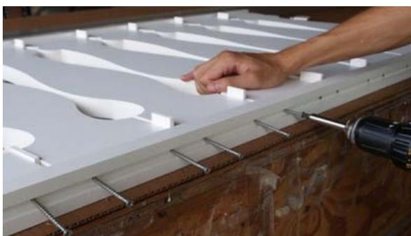
Rotate the Cap Rail and the screws 90 degrees. Be sure the channel is facing out. Fasten the first screw into the baluster nearest the square corner being sure you have proper end spacing and alignment to the square corner. Go to the other end and establish proper end spacing then install one screw. With a screw at each end holding everything in alignment screw the remaining screws in until their heads pull flush. Now flip baluster assembly 180 degrees and repeat for other Cap Rail.
