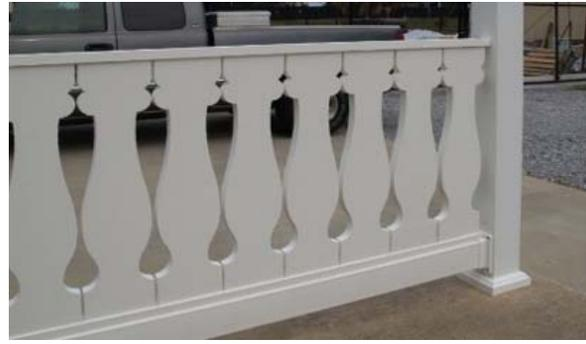
Set the baluster assembly on the bottom rail. If gaps appear, adjust the shims under the rail to make everything level. If any adhesive squeezes out let it stiffen some before removing with a sharp knife. If you use epoxy, it is best to trim any squeeze out before the epoxy fully hardens.
