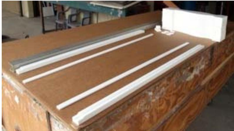
Set up a flat work surface to assemble the Balusters to the Cap Rail. Be sure it is longer than the longest section you will need to assemble. Plywood or a flat door on saw horses is acceptable. The above picture shows the aluminum insert being used as a straight edge. Also pictured are the top and bottom Cap Rail. The Durabrac balusters stacked for assembly. Two long 1/4" thick shims used to raise the balusters to the center of the Cap Rail.
